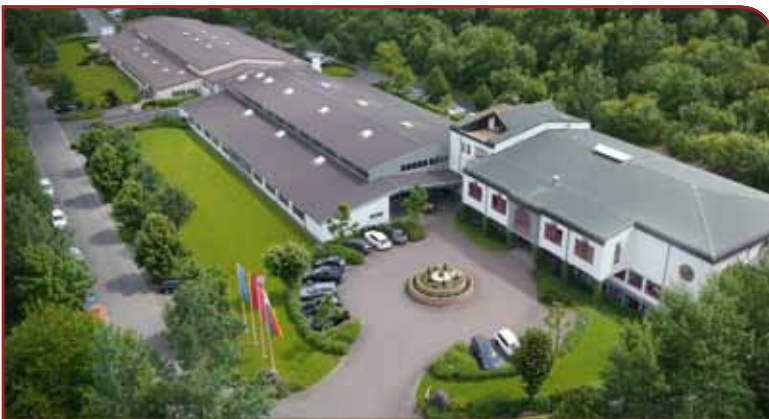
Plant Eiterfeld (36132 Eiterfeld, Hesse) total space: approx. 52,000 m 2
