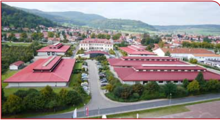
Plant Dermbach (36466 Dermbach, Thuringia) total space: approx. 35,600 m 2
