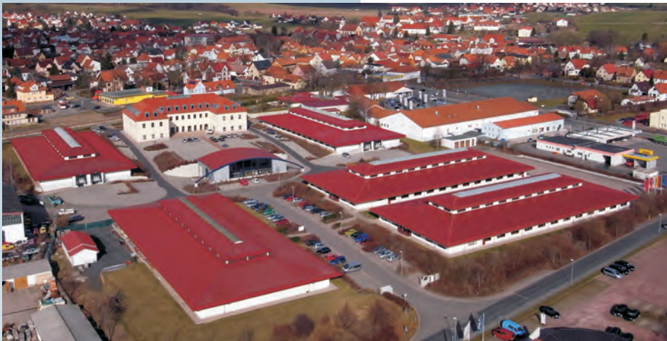
Dermbach (Thuringia) factory sized approx. 14,000 m 2 production, warehouse and office space
